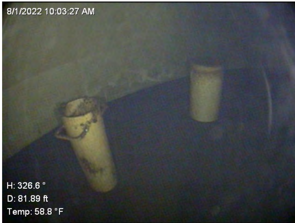
Inlet outlet Pipe
