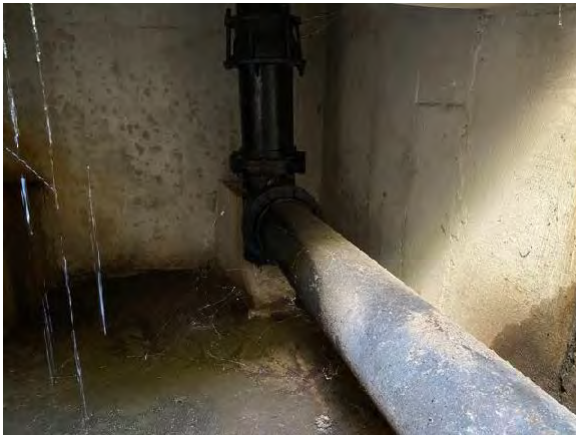
Vault/Pump house piping coating condition Vault area free of standing water
