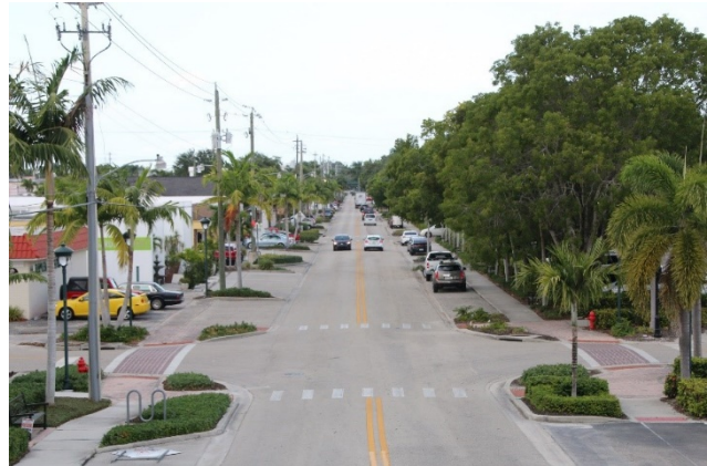
VHB photo of curb extensions
