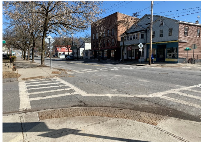
VHB photo of high-visibility crosswalk
