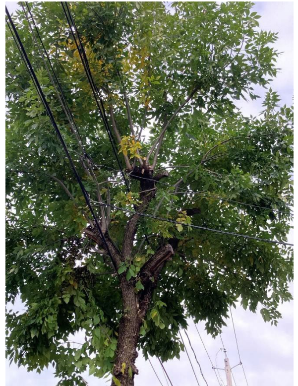
Photograph 3. Tree in Ballston Spa that conflicts with power lines. Tree pruning done to minimize contact with power lines can decrease tree health and structure.
