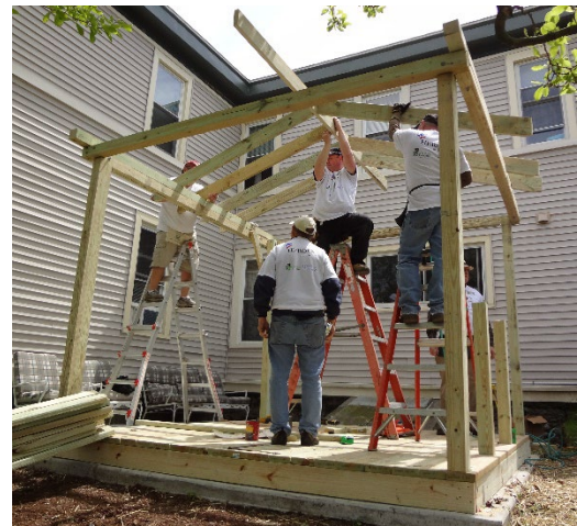
Rotary volunteers working for Rebuilding Together constructing a gazebo for the veteran's home on Church Ave.
