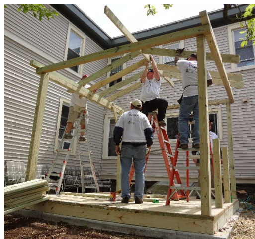
Rotary volunteers working for Rebuilding Together constructing a gazebo for the veteran’s home on Church Ave.
